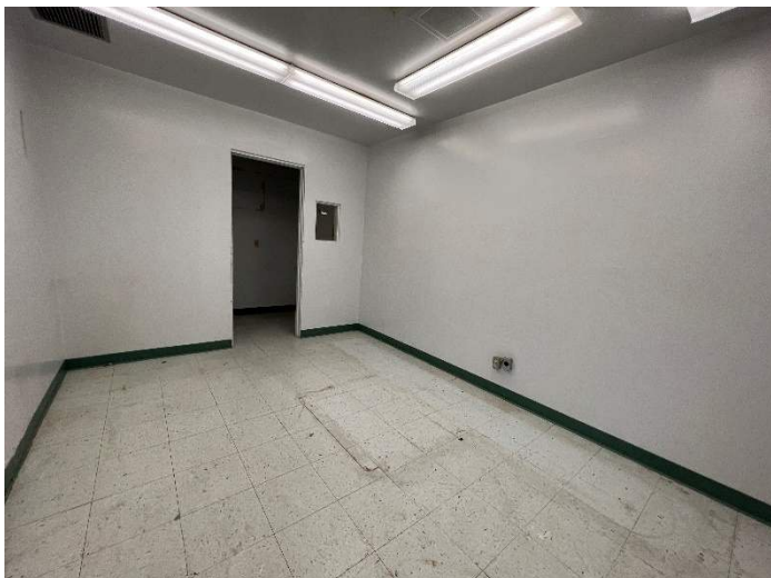
Former X-Ray Room
