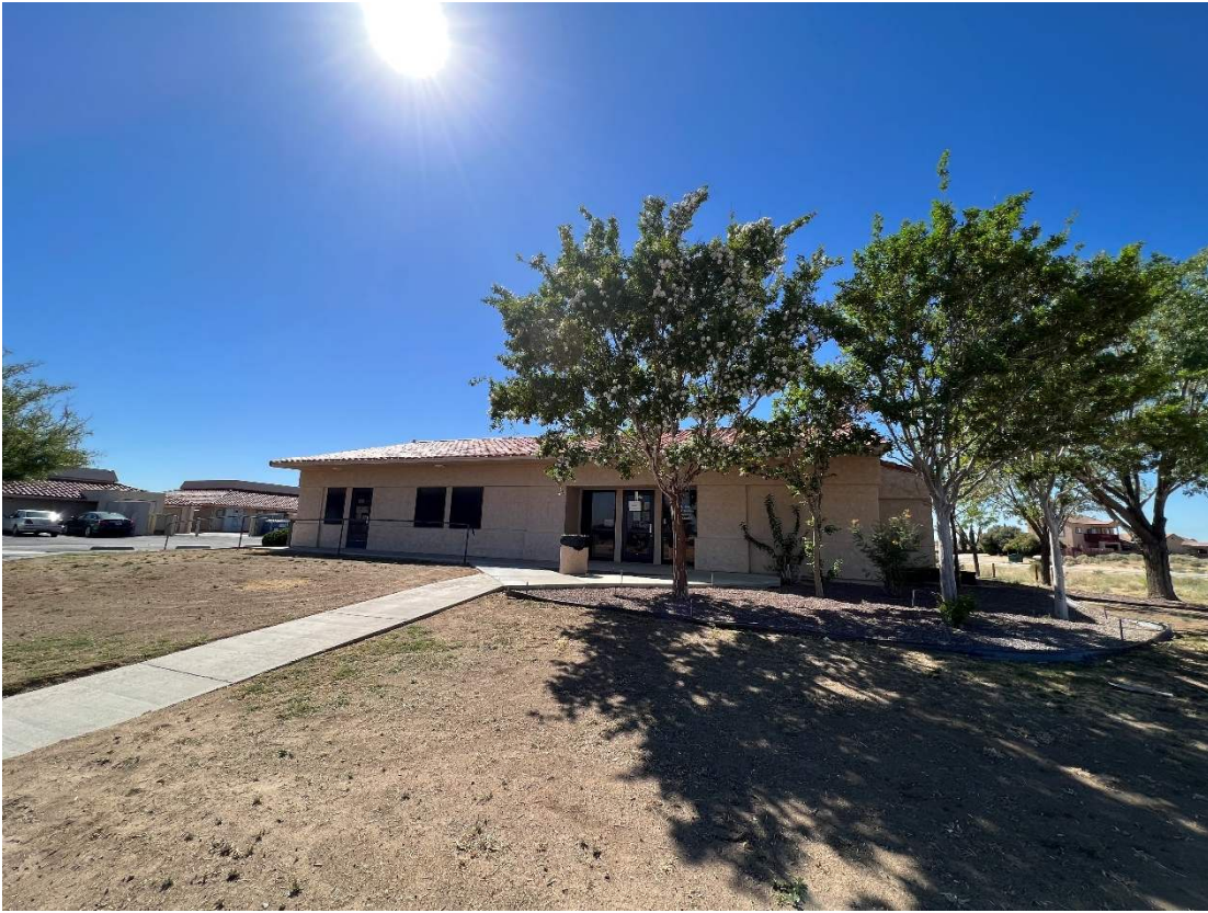
Front View of 9278 N. Loop Blvd. Looking Southeast
