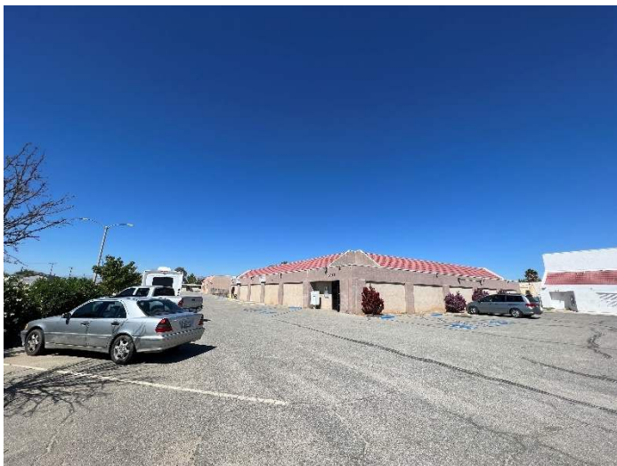
Looking West from Southeast Corner of Property
