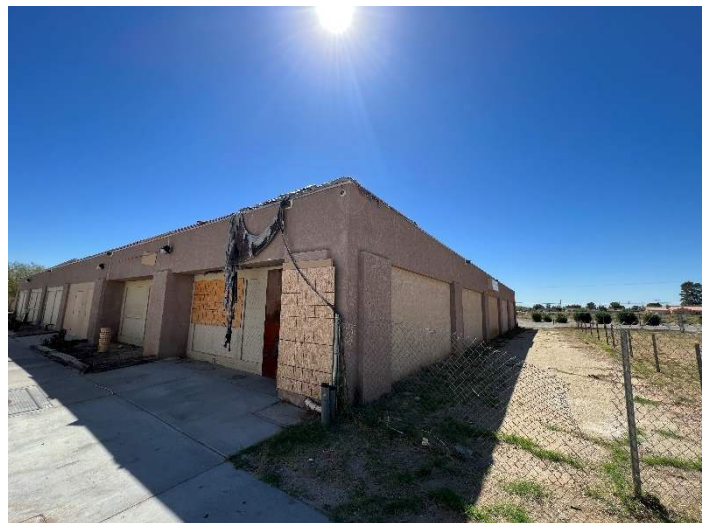
Looking Southeast from Northwest Corner of Property
