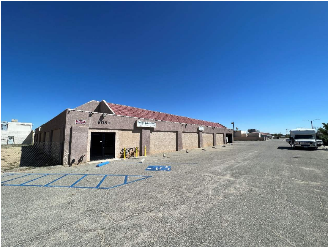
Looking Northeast from Southwest Corner of Property
