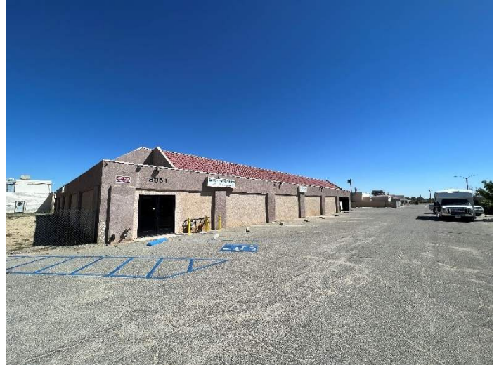
Looking Northeast from Southwest Corner of Property
